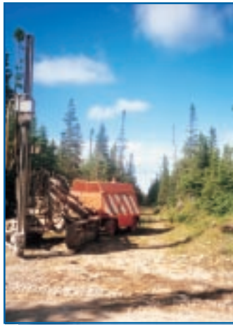
Seismic Shot Hole Drilling
