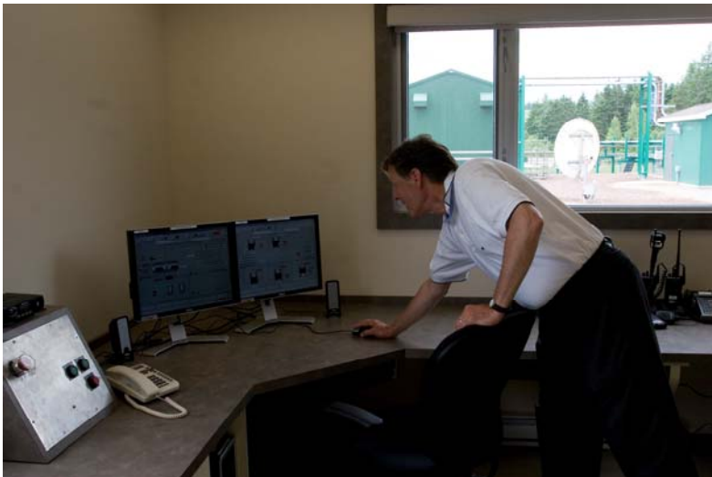
Doug Bailey, Production Operations Manager at the Gas Plant Control Room
