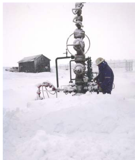
Operator working on a well head.
