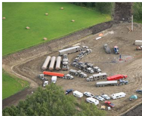
GasFrac equipment at a typical wellsite
