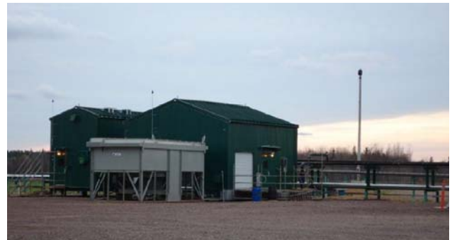
Field Inlet Compressor and Process Building
